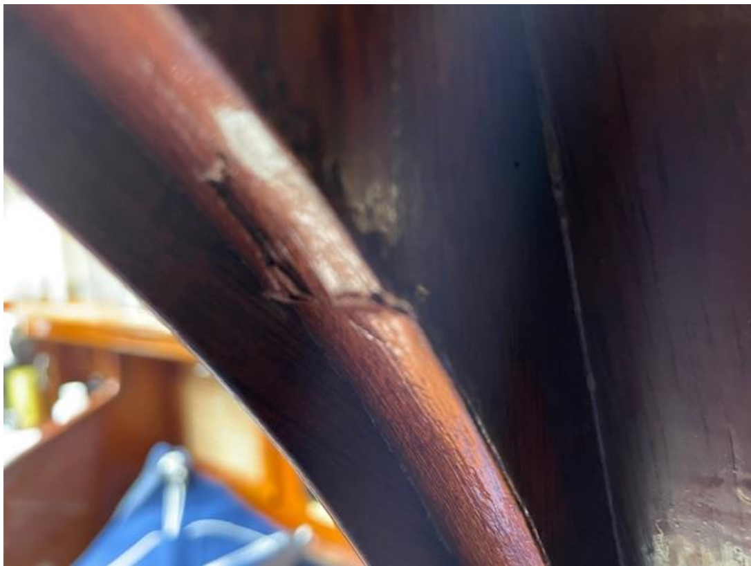
The cracked list on the port side of the main bulkhead
