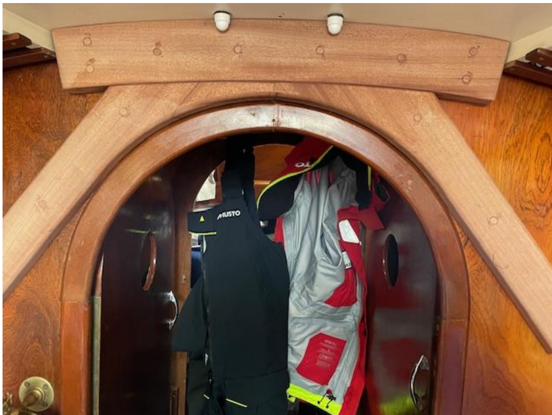
The reinforcement as seen inside the cabin. (Trintella 1-BN321-Castor Spica)
