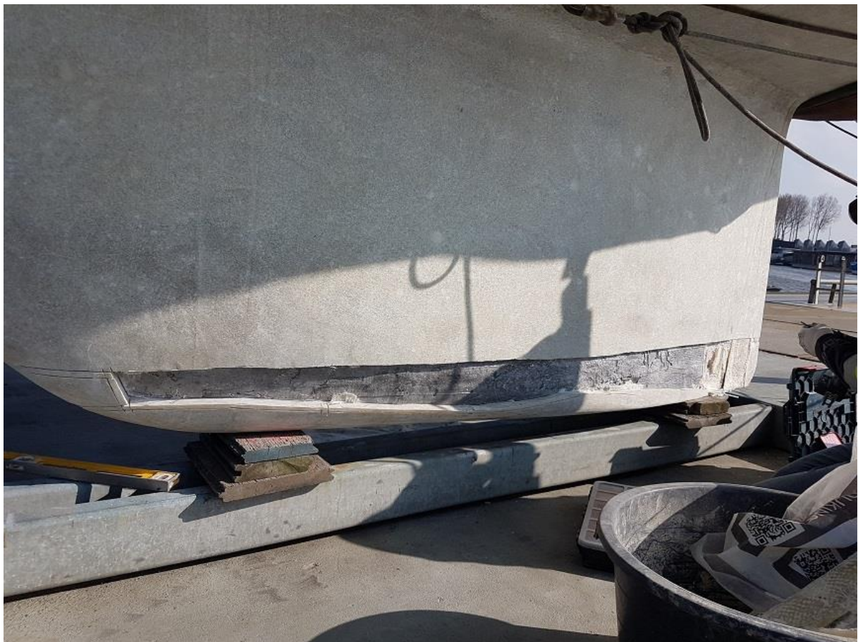
Removing the polyester 12 cm above the future cut line in the lead
