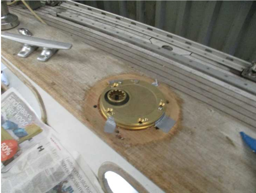
New winch platform
