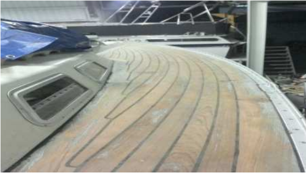
Fig. 19 Ready for mounting the fitting
