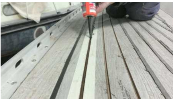
Fig. 16 Taped along the grooves, and caulking ahead of you
