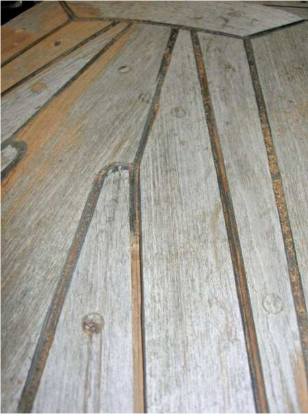
Fig. 12 First groove routed, and a sharp turn visible
