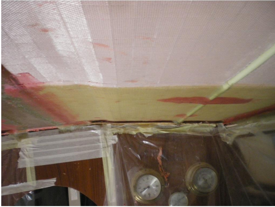
Reinforcement of the cabin roof from the inside
